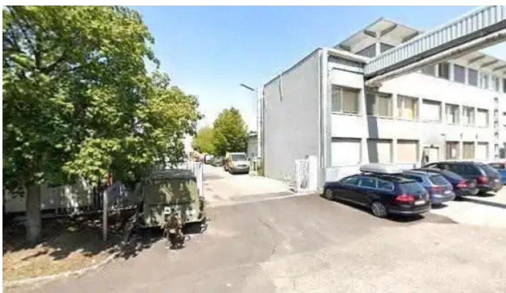
Neveon austria street view 360deg fotos
