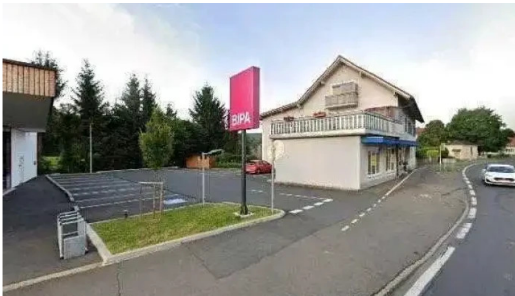
Smatrics ladestation alle
