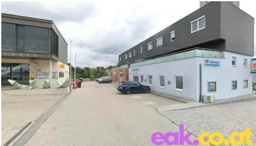
Ecarup charging station eberstalzell
